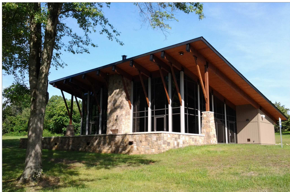
The UT Arboretum Auditorium features nearly 2,000 square feet of open floor space.
